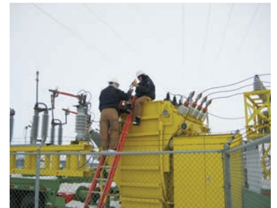
HCE Crews setting up the mobile substation.
